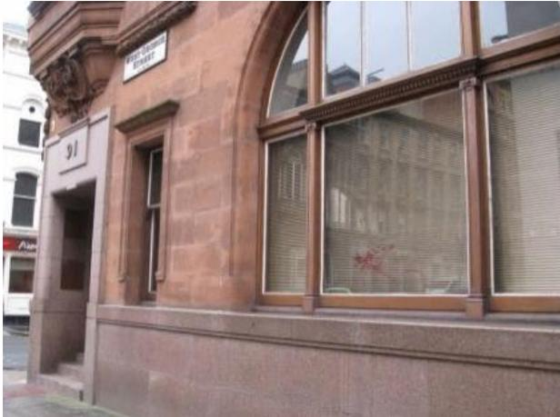
Opposite this, No 91, another former bank was designed in a very characteristic way for banks in Glasgow, with a base of pink Peterhead Granite and upper storeys of red sandstone. The granite contains pink feldspars, clear quartz and dark mica, and many small patches of black and white xenoliths.
