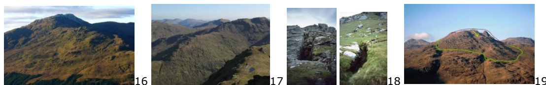
16 - Ben Donich N ridge seen across Glen Croe - the RSF slump has almost reached the forest 17 - Ben Donich N ridge seen from Beinn an Lochain - headscarp dotted (image courtesy Bert Barnett) 18 - tension fractures on Ben Donich upper north ridge - the fissures become hazardous if overgrown 19 - The Cobbler from The Brack - the short and longer-travelled RSF elements have left 3 fang peaks behind; red envelope suggests original summit plateau, as at Beinn Narnain (rear right)
