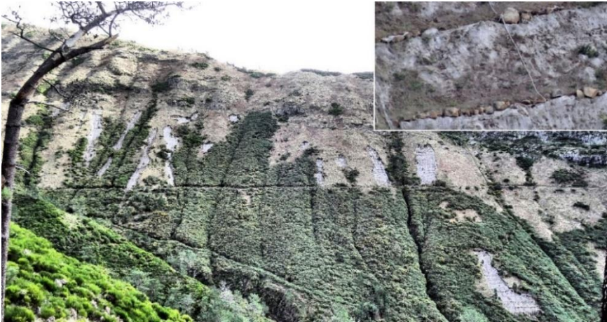
Fig. 21. Steep west facing slope of Lombo do Buxo scarred by landslips. Inset is an enlargement of a scar to illustrate the boulders securing netting
