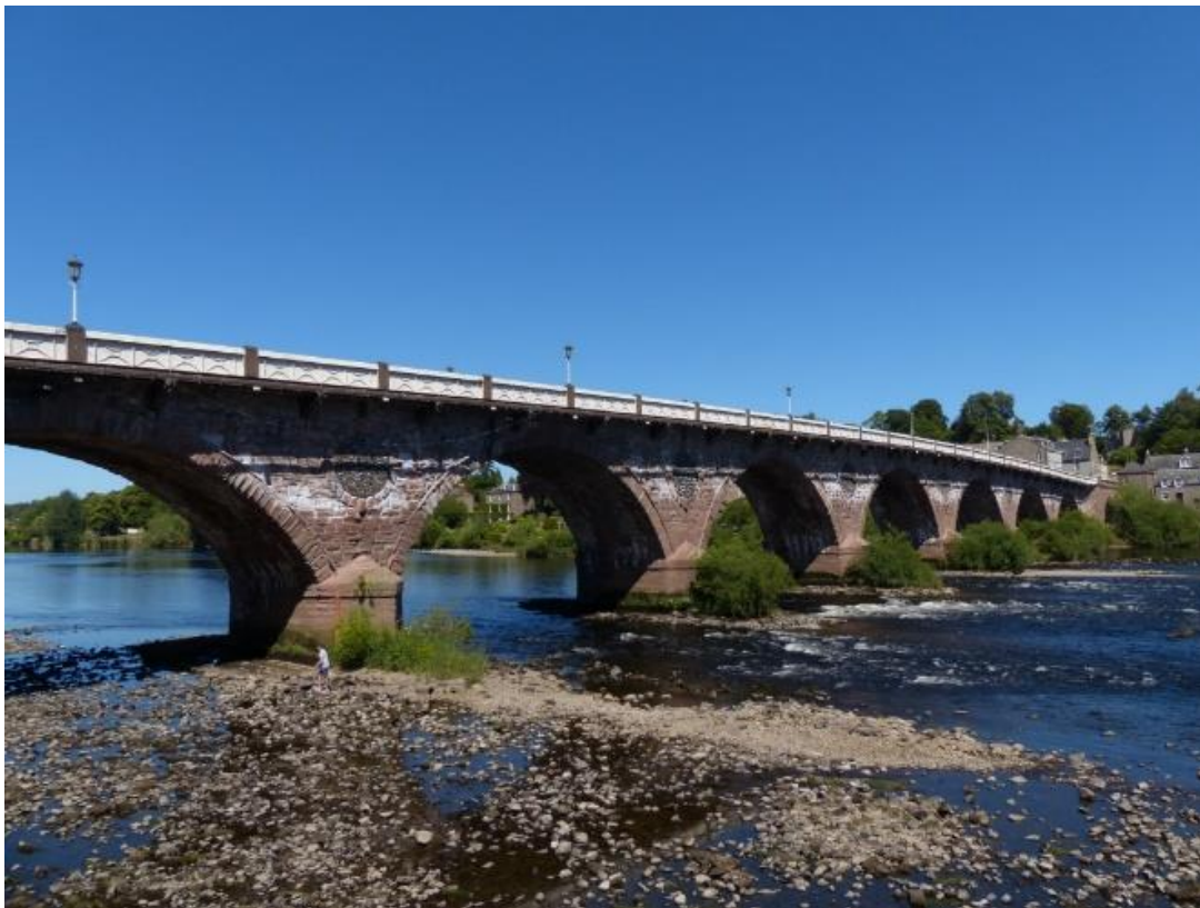
Smeaton Bridge (Locality 16.5). The columns are made of Scone sandstone & the spandrels (the circular inserts) of basalt. Bill Gray
