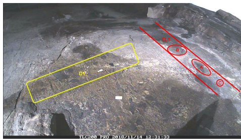
Frame from time-lapse camera showing areas of condensation drips (red) and drips from roof leaks (yellow). Photo courtesy of Historic Environment Scotland.
