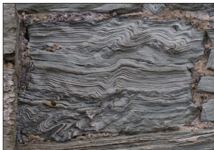
Fig. 17. Highly folded green mica schist of the South Stack Group, used as building blocks at Breakwater Park, Holy Island (Bill Gray)
