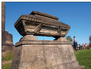
Fig. 10. Rev. Dr. Thomas Brown's tomb has been badly corroded by acid rain.
