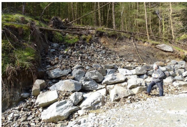
Fig. 11. Rare collapse of an unusually thick deposit of unconsolidated drift. The large boulders were placed to protect the road from any further slippage.
