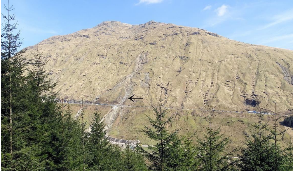
Fig. 8. The slopes of Beinn Leubhean above the A73(T) in Glen Croe. Note the scar (see arrow) left by a recent landslide that closed both the main road and the Old Military Road. There is a risk of further landslips across the entire width illustrated, but especially from the slopes on the left-hand half side of the photograph.
