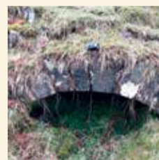
Old Lime Kiln, Banton burn
