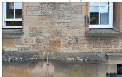
Fig. 14. Bower Building. Ashlar blocks below, snecked pattern above.
