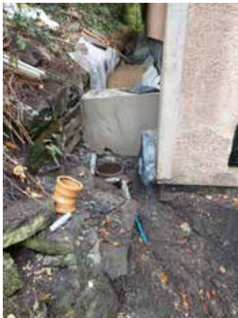
Drainage and tanking works on the south elevation
