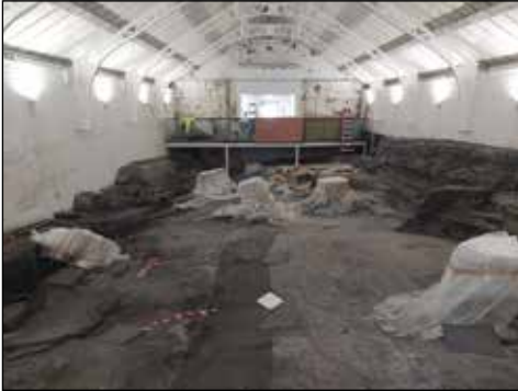
Old lighting removed and roof structure painted
