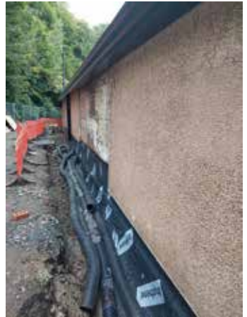
Drainage and tanking works on north elevation
